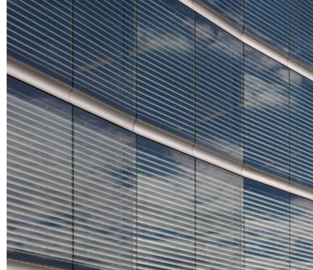
▶ The special external venetian blind model supports the design concept and considerably enhances comfort inside the building.
